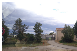
RN 7, la STEP, station d'épuration
